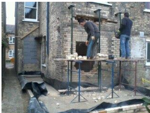
Demolition work begins at Judith Green’s home.
