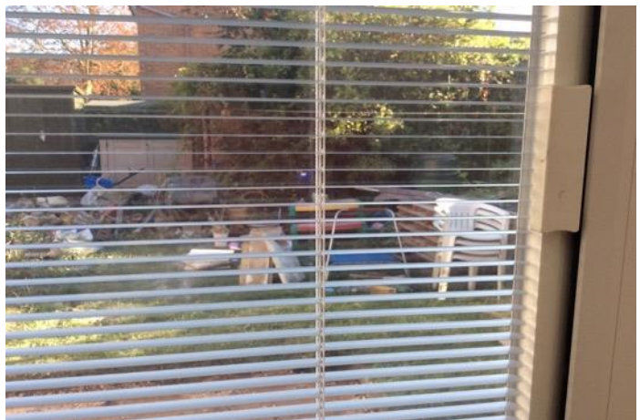
Blinds in-between the double-glazing panes
